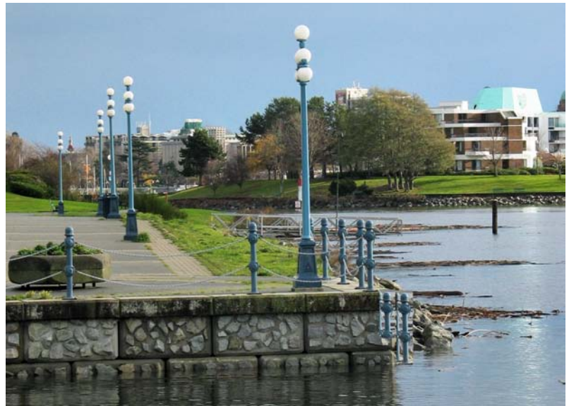
Fig. 2. Location of the marina restaurant building at high tide of 2.68 m. The water is 1.07 m (3.5 ft) below the surface of the walkway. At the highest tide the water is 0.55 m (1.8 ft) below the walkway.
